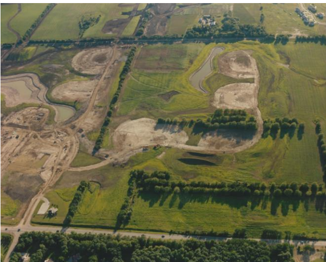
An early view of Prairie Crossing (courtesy of Aerial Images) with excavations of Lake Aldo Leopold and Sanctuary Pond along with the Osage Orange, Village Green, and Prairie Trail areas.
